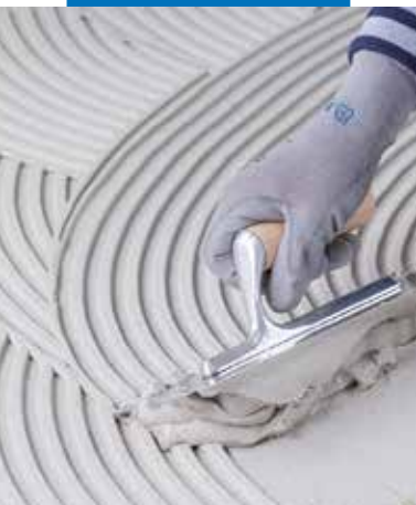
Spreading Adesilex P9 white
