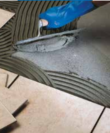
Installation of single-fired tile on floor
