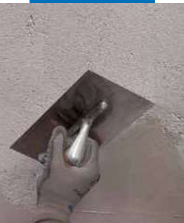
Application of Mape-Antique FC Civile
