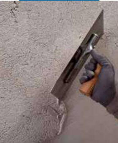
Application of Mape-Antique FC Civile
