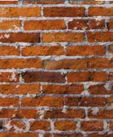
Brick wall after removing the deteriorated render
