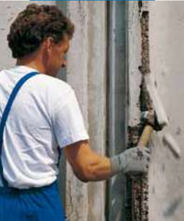
Demolition of degraded concrete
