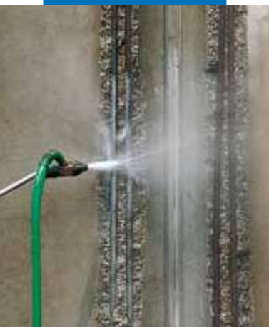
Cleaning reinforcing rods
