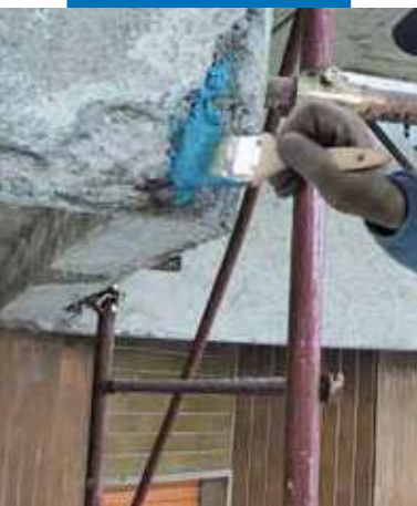
Applying Mapefer 1K with a brush on reinforcing rods on a reinforced concrete balcony
