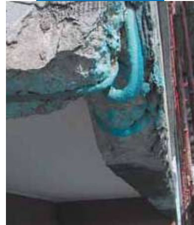
Reinforcing rods on the front side of a balcony treated with Mapefer 1K
