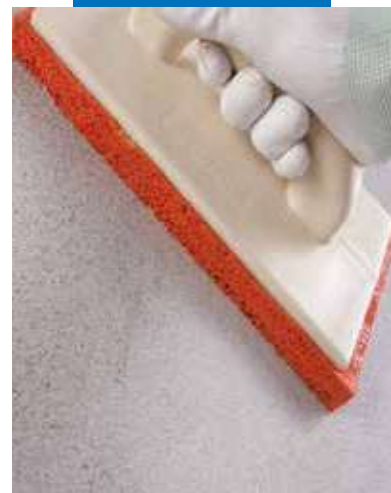
Finishing off the surface of the smoothing and levelling layer with a sponge float
