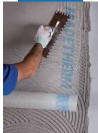
Application of a reinforced smoothing and levelling layer by embedding Mapetherm Net
