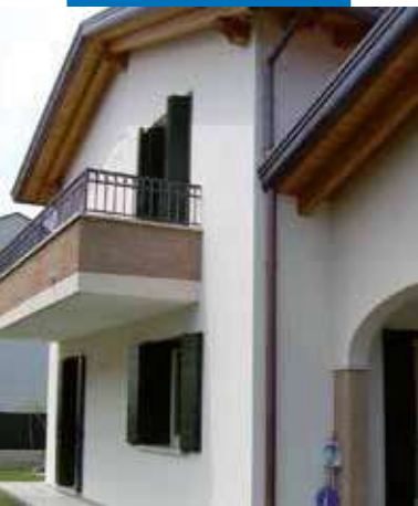
Reggio Emilia - Italy - Work on a private home using Mapetherm AR1 GG
