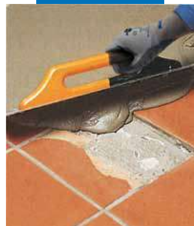
Filling holes with Nivorapid
