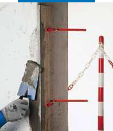
Repairing vertical arrise with Nivorapid
