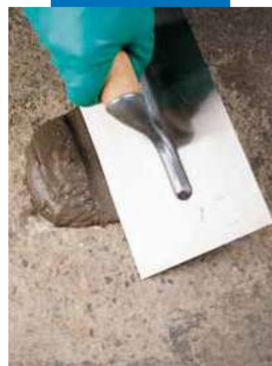
Repairing horizontal arrises with Nivorapid
