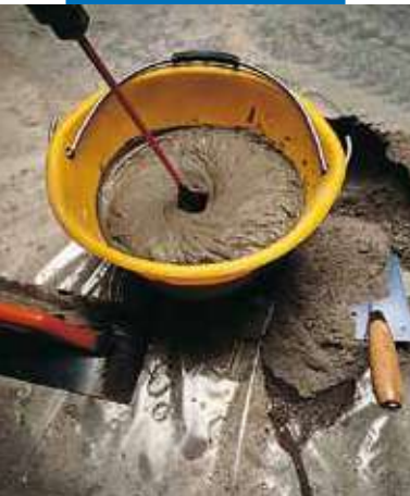
Nivorapid mixed with mechanical mixer
