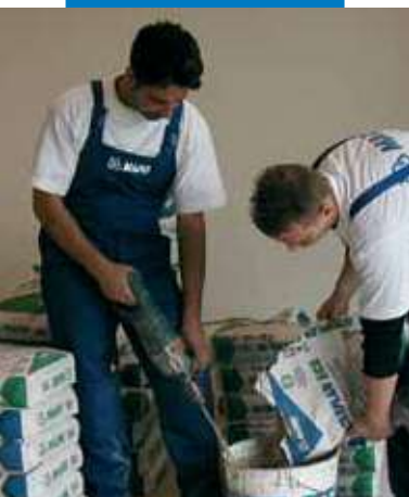
Mixing Ultraplan Eco - Mirabello kindergarten - Cantù (Como) - Italy
