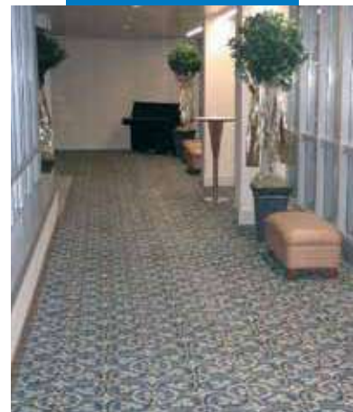
Carpet laid on a hotel corridor after levelling with Ultraplan Eco - Hotel Renaissance - Austria
