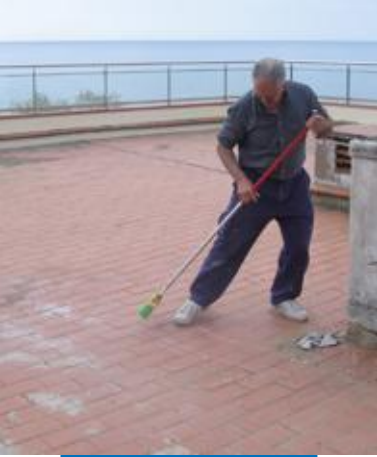
Cleaning a substrate before applying Aquaflex Roof
