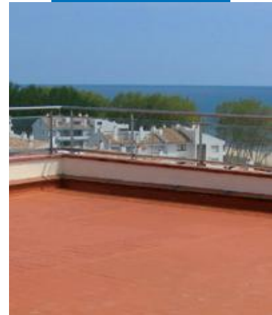
Paving slab waterproofed with Aquaflex Roof
