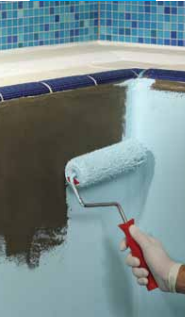
Application of Elastocolor Waterproof with a roller
