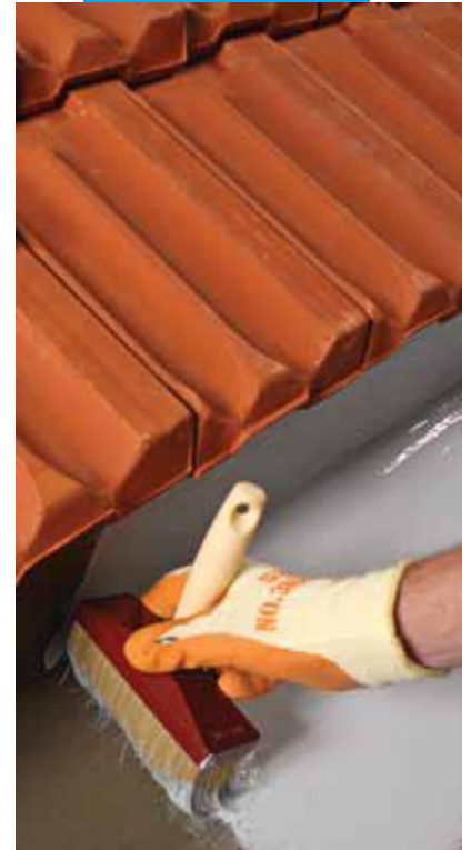
Example of a gutter waterproofed with Mapelastich Smart and coated with Elastocolor Waterproof
