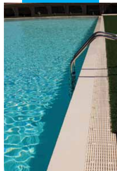
Detail view of a swimming pool dressed with Elastocolor Waterproof
