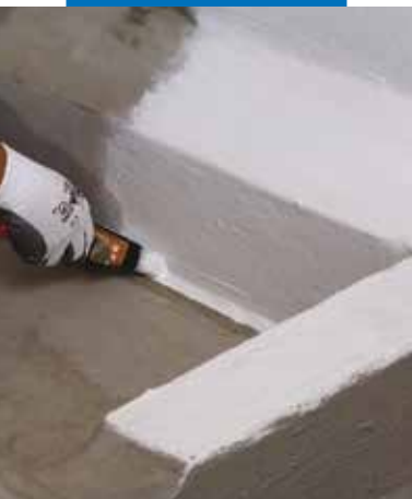
Triblock P applied to blend in the joint between a floor slab and a vertical wall
