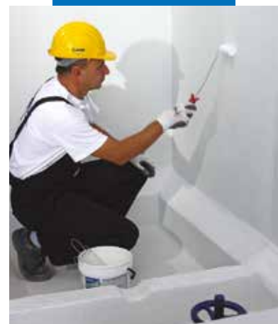
Application of Triblock P by roller
