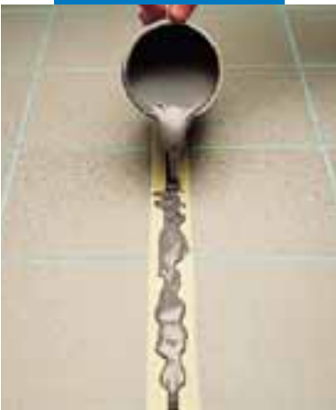
Filling the joint with Mapeflex PU21
