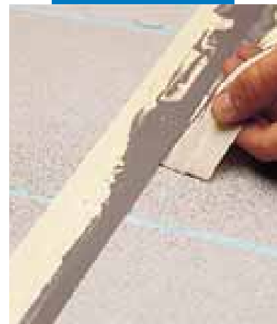
Removing the masking tape from the joint
