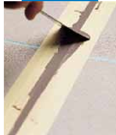
Smoothing the joint
