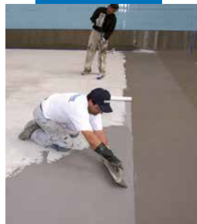
Waterproofing a swimming pool with Mapelastic
