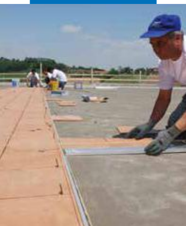
Installing ceramic with Kerabond + Isolastic
