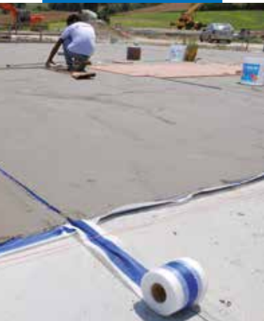
Waterproofing screeds with Mapelastic and Mapeband
