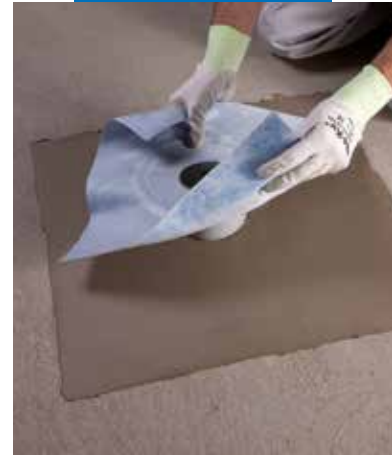
Application of Drain Vertical on Mapelastic
