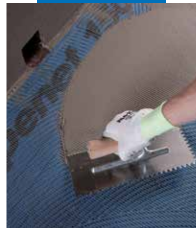
Laying Mapelastic on Mapetex 150
