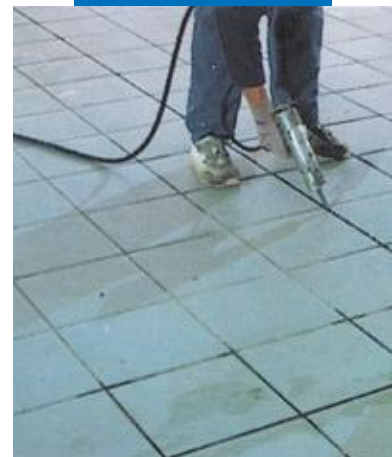
Sealing ceramic tile floor with Mapesil AC
