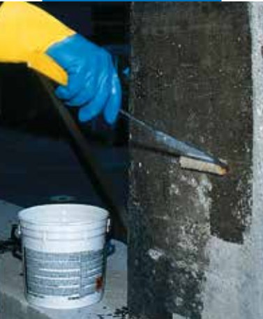
Applying MapeWrap 31 with a roller on the still fresh MapeWrap 11 (or MapeWrap 12)
