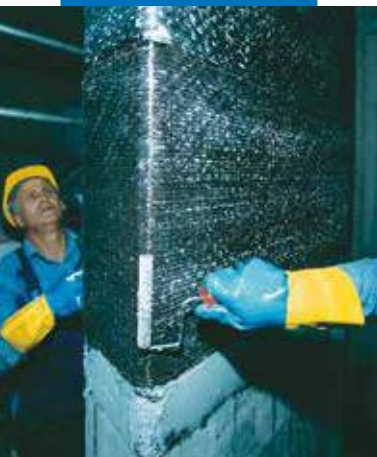
Applying pressure on the fabric with the Roller for MapeWrap so that MapeWrap 31 can penetrate well into the fabric
