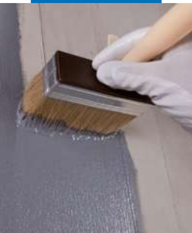
Application of Eco Prim Grip on concrete by brush
