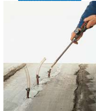
Restoring horizontal structure by injection with Epojet
