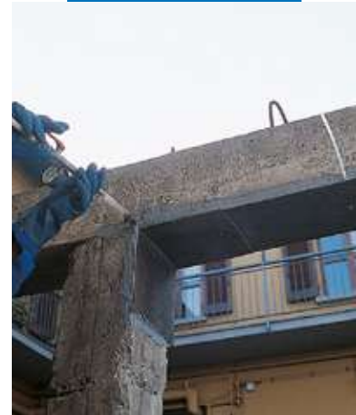
Repairing beam with injection of Epojet
