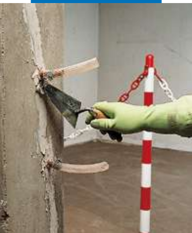
Fixing injection tubes with Adesilex PG1
