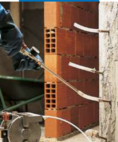
Injecting Epojet to a fissured pillar
