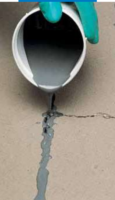
Repairing a crack in cement screed with Eporip
