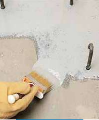
Applying Eporip by brush on construction joint
