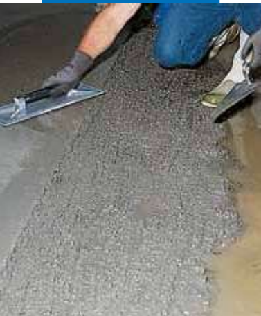
Screeding with mortar admixed with Idrosilex Liquid
