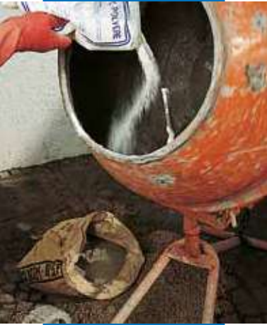
Preparing waterproof mortar admixed with Idrosilex Powder
