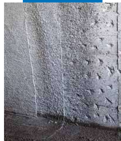
Applying mortar admixed with Idrosilex over concrete roughened with a bush hammer
