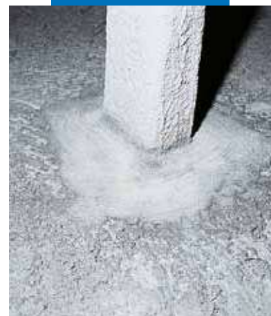
Column waterproofed with Idrosilex
