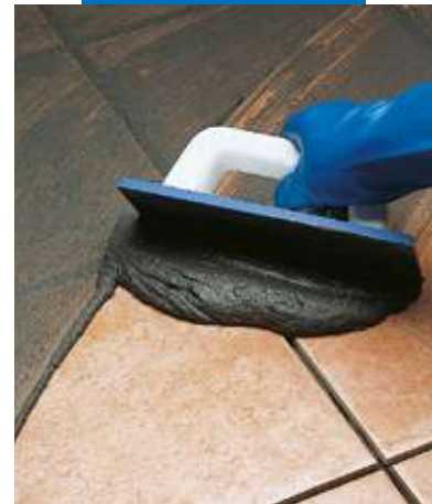
Grouting single-fired tiles with a float
