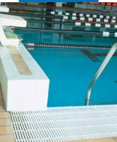
An example of an installation of mosaics with Keracrete in a swimming pool
