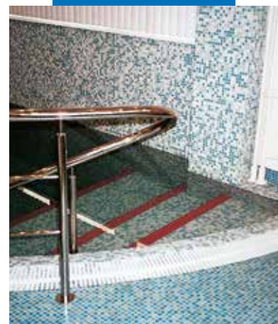
Laying glass mosaics
