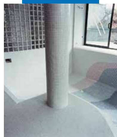
Installation of mosaics
