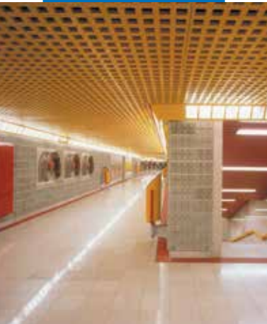
An example of an installation of Granitello in underground - Linea 3 - Milan (Italy)
