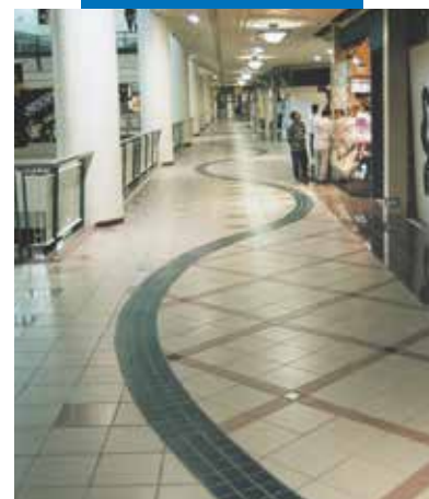
An example of an installation of ceramic tile in a mall - Filinvest Festival Superhall - Manila (Philippines)
