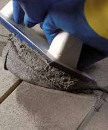
Spreading Kerapoxy CQ using a MAPEI float
