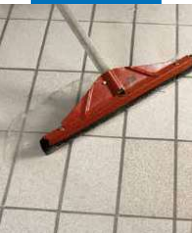
Removing excess liquid using a rubber squeegee
