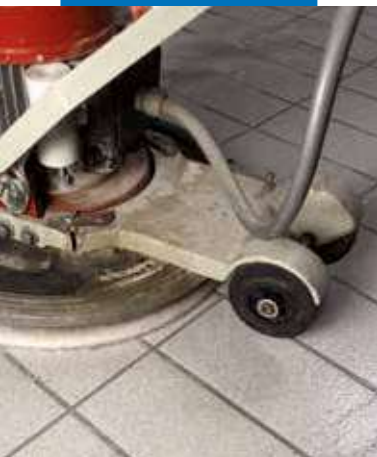
Cleaning the surface with water and single-head rotary machine with special abrasive felt discs, such as "Scotch-Brite®"
