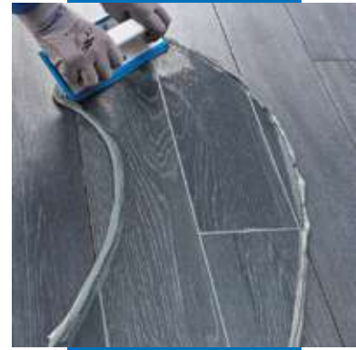
Spreading Kerapoxy Design on wood-effect porcelain floor tiles with a rubber trowel
