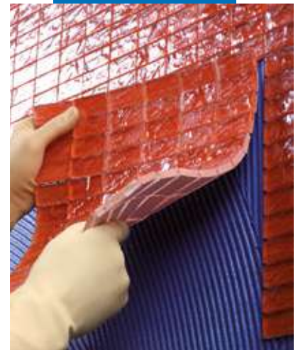
Laying glass mosaic with Kerapoxy Design on wall
