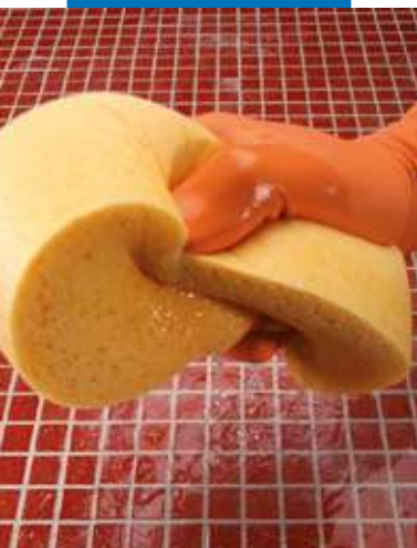
Wetting the surface of the grout before cleaning
