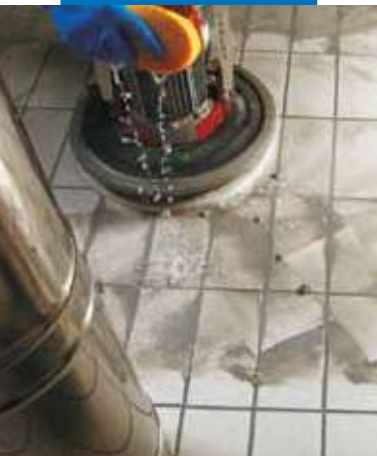
Cleaning off Kerapoxy P with water and a single head rotary machine with Scotch-Brite®
