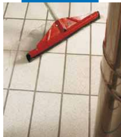
Cleaning off the flooring surface with a rubber raker
