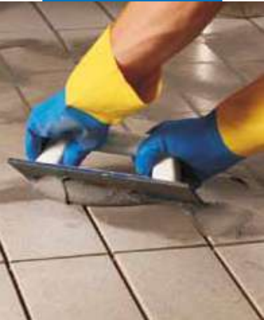
Grouting floor joints with a rubber trowel
