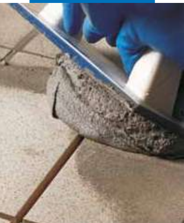
Grouting floor joints with a rubber trowel
