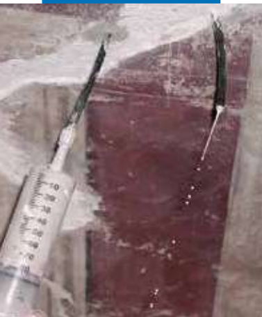
Injecting Mape-Antique F21 into a frescoed wall
