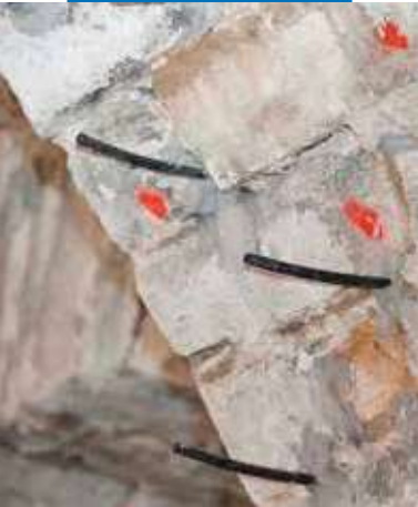
Detailed view of how the injection tubes are fastened in place
