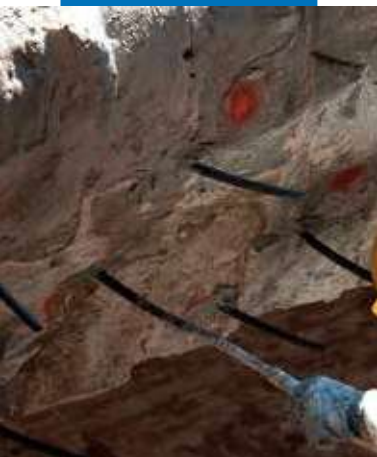
Injecting Mape-Antique F21 into a stone masonry
