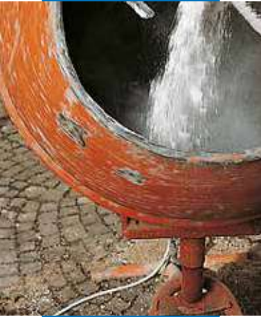
Mixing mortar on site with locally-sourced aggregates
