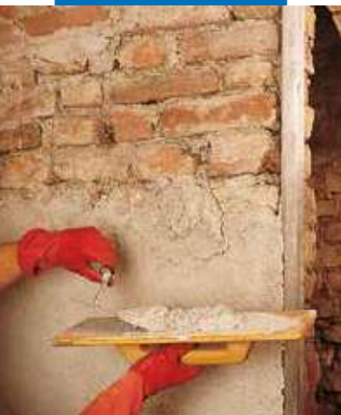
Application of de-humidifying render mix on site
