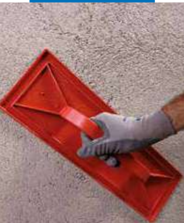
Levelling the surface of Mape-Antique MC
