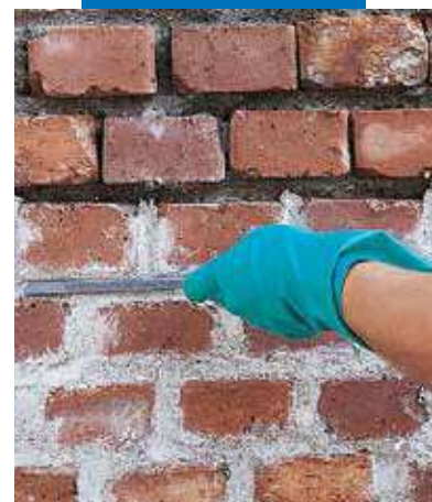
Finishing mortared joints pointed with Mape-Antique MC
