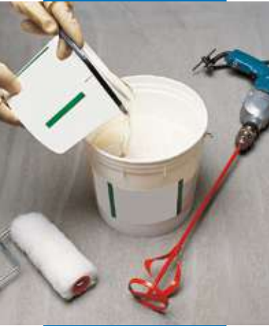
Mixing component B with component A
