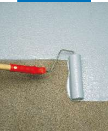
Applying Mapecoat I 24 with roller
