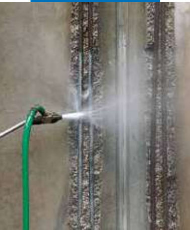
Cleaning reinforcing rods with hydro-sandblasting
