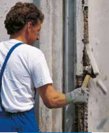
Demolition of degraded concrete
