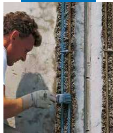
Application of Mapefer
