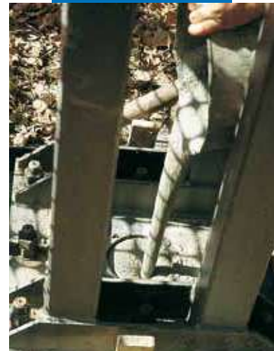
Anchoring of structural steel work with Mapecoll
