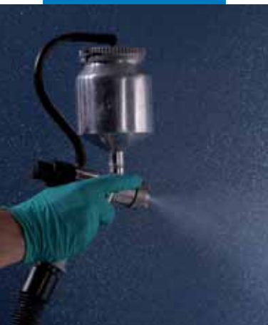
Finishing off Silancolor Tonachino with Mapelux Lucida and MapeGlitter Silver
