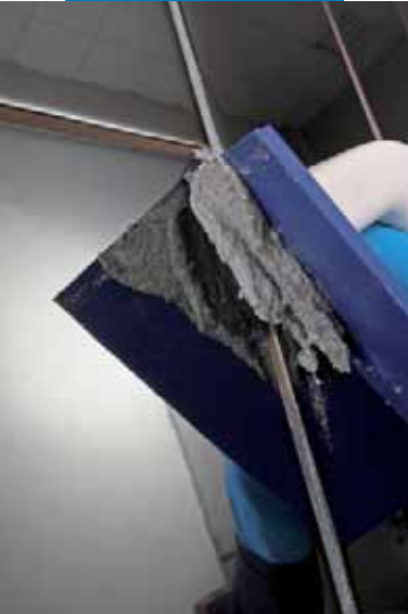
Grouting joints with Kerapoxy Design and MapeGlitter Silver
