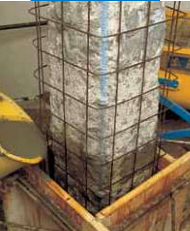
Pouring into a formwork
