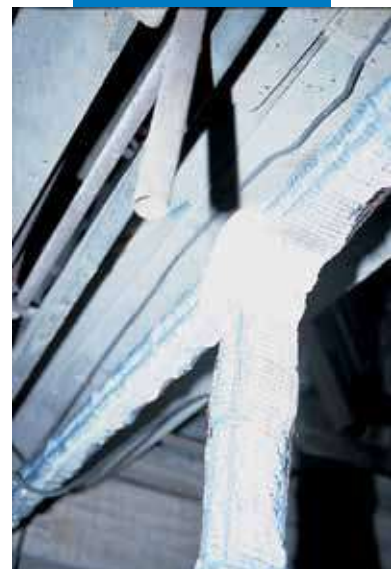
Deteriorated concrete structure
