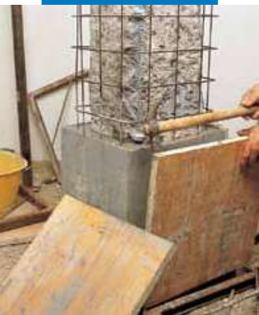
Removing wooden formwork
