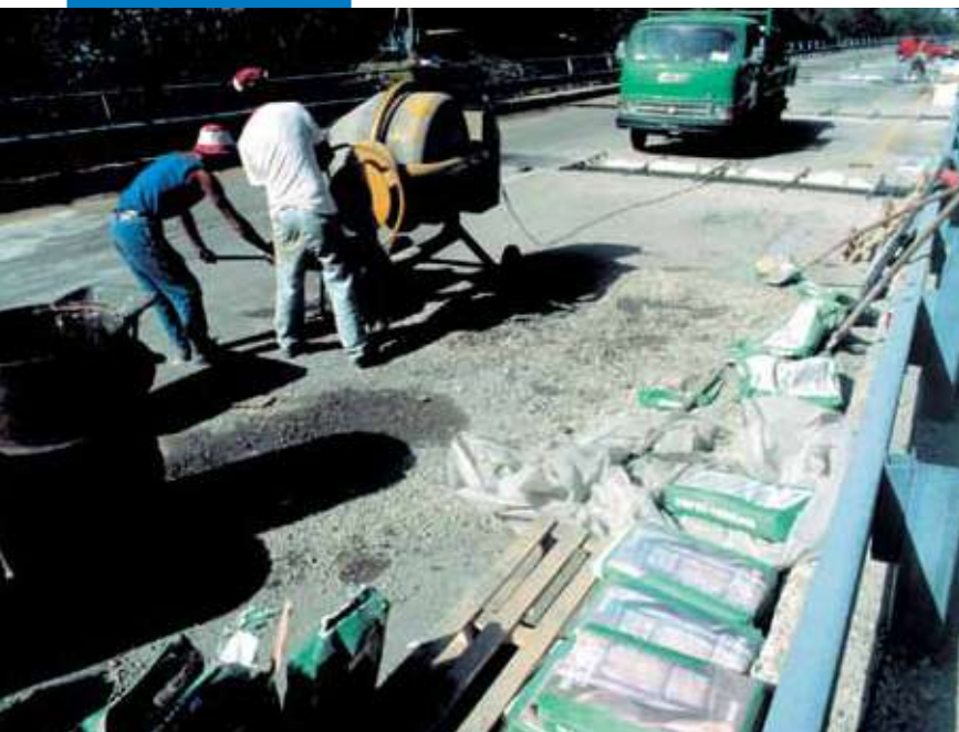
Reforming road joints
