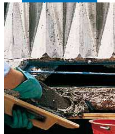
Repairing a balcony with Mapegrout T40
