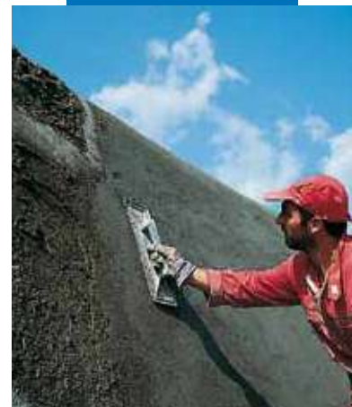
Finishing of Mapegrout T40
