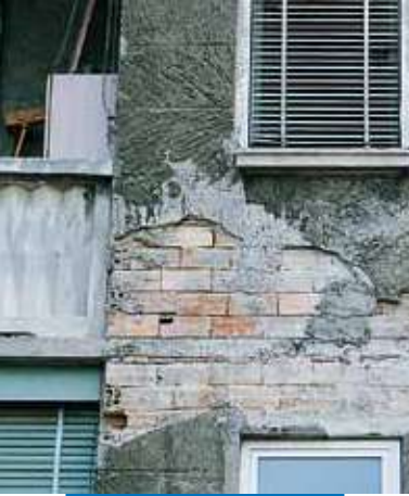
Degraded building façade in need of repair
