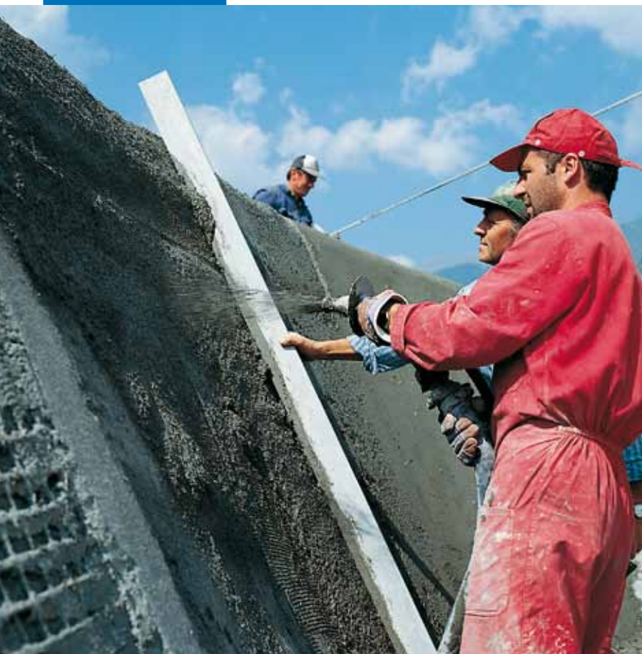
Spray application of Mapegrout T40
