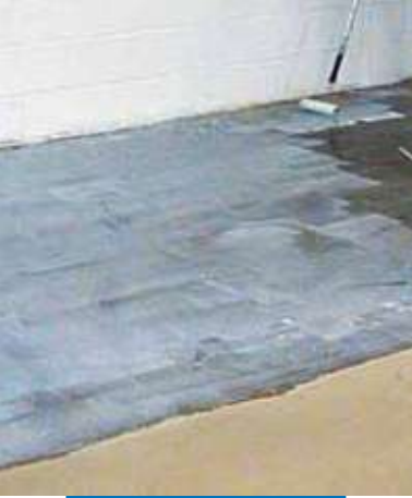
Application of Mapeprim SP
