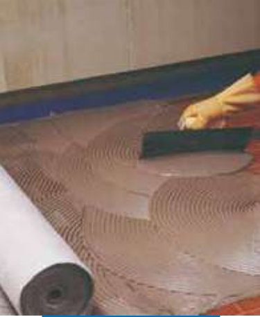
Application of the first layer of Mapelastick, and successive laying of Mapetex Sel
