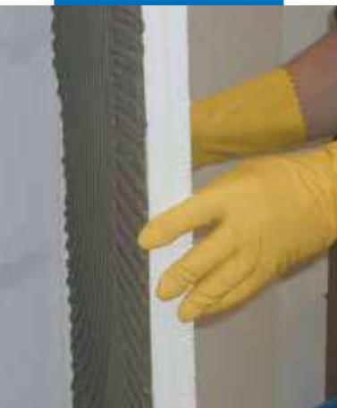
Installing the insulating panels
