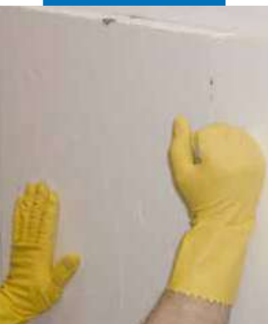
Applying pressure on the panels once they have been installed. This is to ensure a good bonding to the surface
