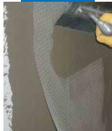
Smoothing insulating panels reinforced with a Fibreglass Mesh drowned into the coat of Mapetherm AR1
