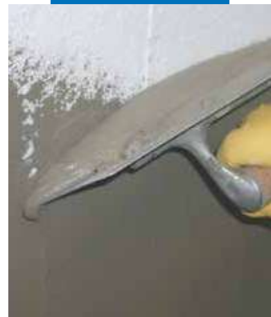
Smoothing insulating panels: spreading the Mapetherm AR1
