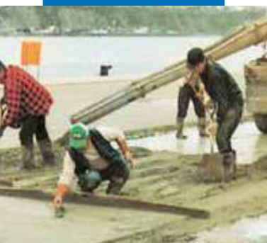
External cementitious screed with Planicrete admix - Vieux Port, Quebec, Canada
