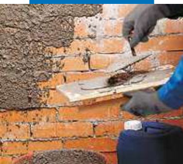
Base-keying mortar layer with Planicrete admix
