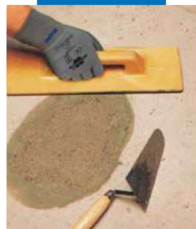
Floor patching: final smoothing
