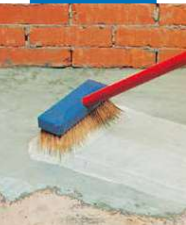
Application of cementitious grout with Planicrete admix
