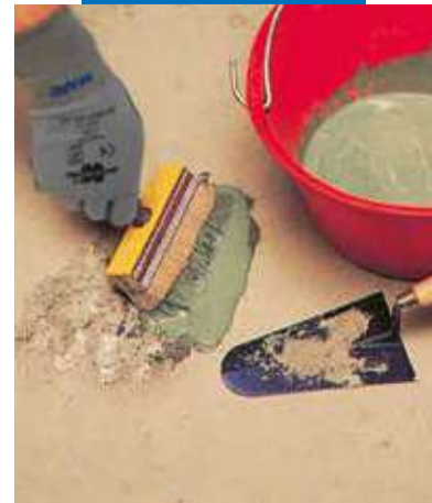
Floor patching: application of slurry
