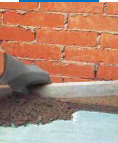
Application of cementitious screed with Planicrete admix
