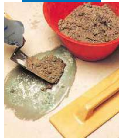
Floor patching: application of mortar
