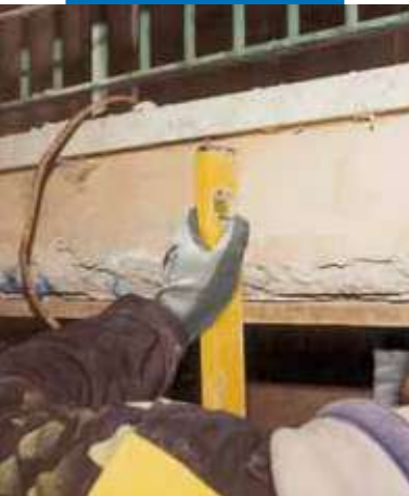
Restoring the front of the concrete slab of a balcony: positioning wooden form work
