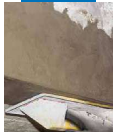
Patch-work of a concrete beam
