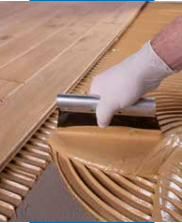
Spreading Ultrabond P990 1K
