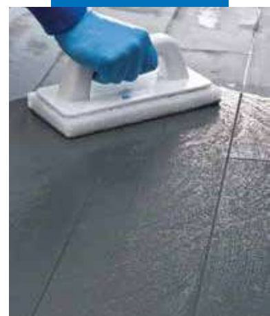
Cleaning the joints with a Scotch-Brite® pad (when the product is semi hardened)
