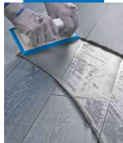
Spreading Ultracolor Plus on wood-effect porcelain floor tiles with a rubber float
