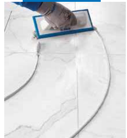
Spreading Ultracolor Plus on marble-effect porcelain floor tiles with a rubber float
