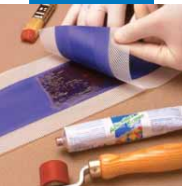
Joining the Mapeband strips
