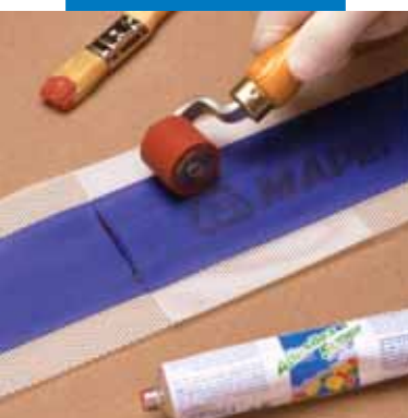
Use a roller to press the joints of the Mapeband strips together
