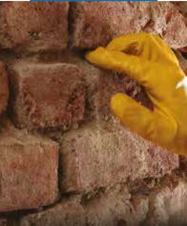
Consolidating the substrate
