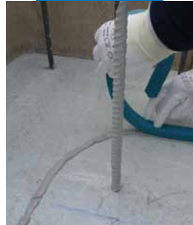
Applying Idrostop Soft on horizontal surfaces
