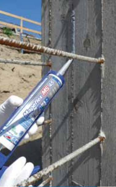
Extruding Mapeflex MS45 prior to applying Idrostop Soft in second pours
