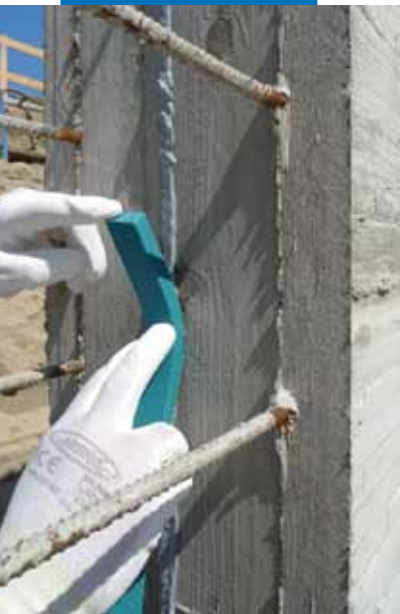
Applying Idrostop Soft on vertical surfaces
