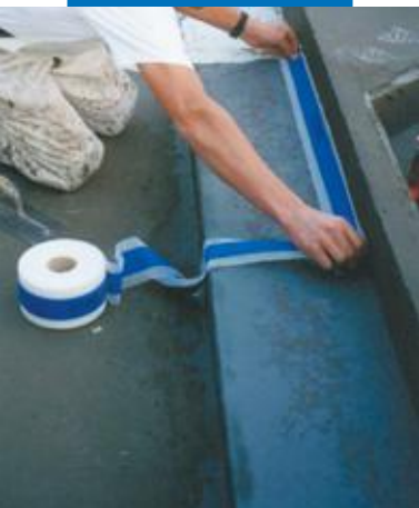
An example of Mapeband waterproofing a corner between the bottom and a side of a bath tub
