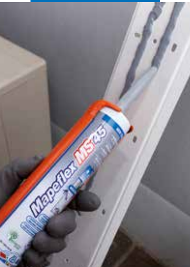
Bonding plastic profiles on a surface outside
