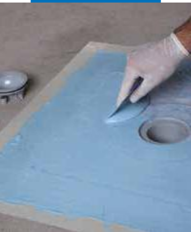
Impregnating Drain Vertical fabric with Mapelastick AquaDefense
