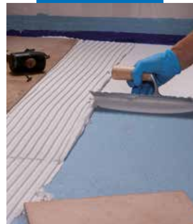
Bonding tiles on Mapelastac AquaDefense
