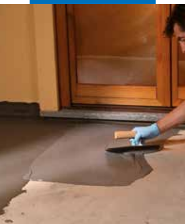
Waterproofing of terraces by trowel
