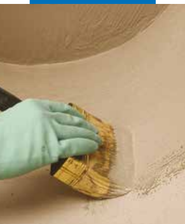
Waterproofing of details by brush
