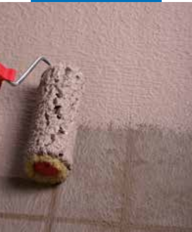
Waterproofing of details by roller
