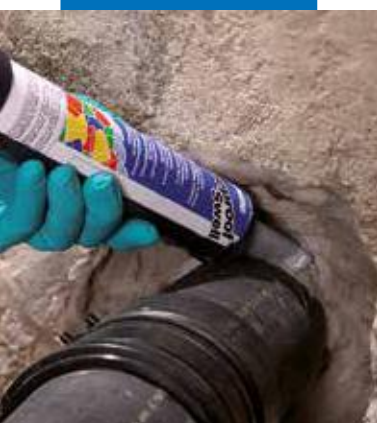
Applying Mapeproof Swell around a pipe
