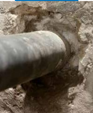
Breaking out structure around a pipe
