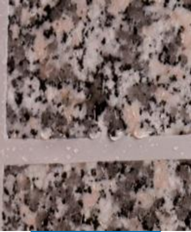
Sealing a butt joint on natural stone
