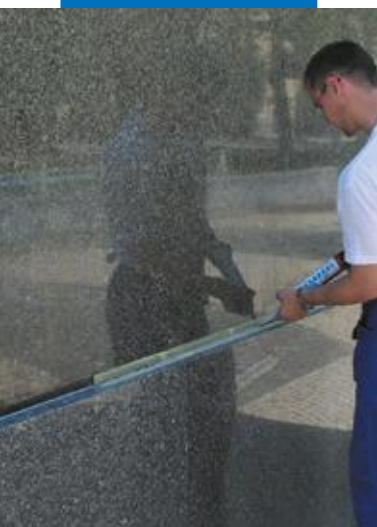
Sealing a façade joint with Mapesil LM
