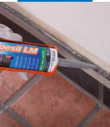
Sealing a fillet joint on natural stone
