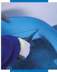
Cut the lower part of Mapesilent Band R to form a 90° angle
