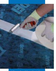
After checking that the sheets of Mapesilent Roll overlap perfectly, seal all overlaps using Mapesilent Tape
