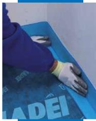
Place the rolls of Mapesilent Band R side by side. Remove the protective film from the back and bond around all the perimeter of the room
