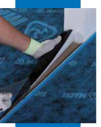
Unroll the sheets of Mapesilent Roll, place it against the bottom of the wall and start laying it with the fibre side (the light-coloured side) underneath. following the longer side of the room. Lay the second sheet at the bottom of the wall, taking care to remove the protective film from the back of the border used to overlap with the adjacent sheet (approximately 5 cm), to guarantee the continuity of the layer
