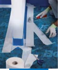
Apply Mapesilent Tape along the overlaps of Mapesilent Band R and Mapesilent Roll and the joints between the various sections of Mapesilent Band R
