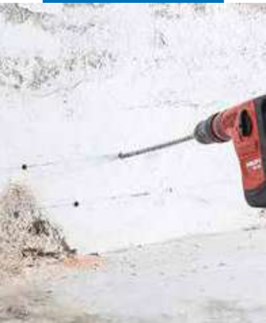
Drilling the holes
