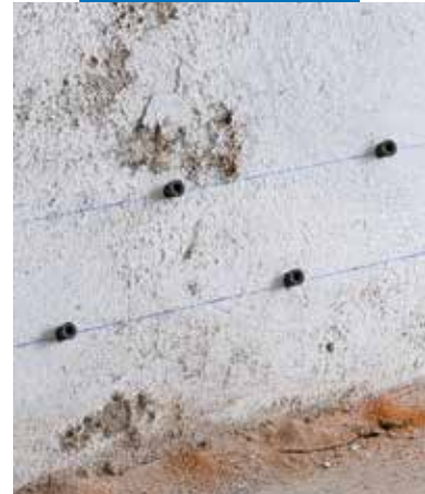
Detail of the staggered rows of holes
