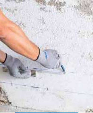
Preparing the holes
