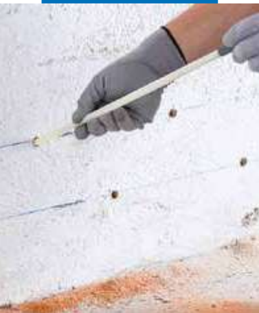
Inserting the injectors in the holes
